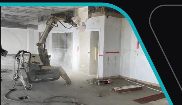
Using demolition robots in tight/restricted access areas is a great way to reduce the amount of HAVS (Hand Arm Vibration syndrome). Keeping the operator at a safe distance controlling the robot that is 10 times more powerful than traditional methods.
